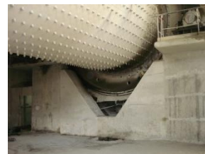
Base foundation survey
